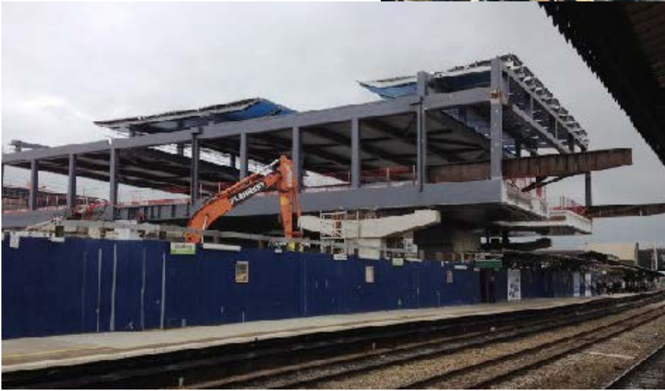
Bridge slide across railway, Reading
