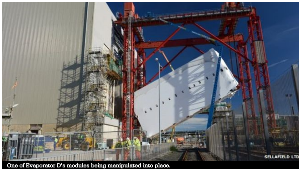
One of Evaporator D's modules being manipulated into place.
