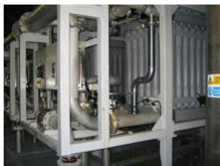
one of the continuous micro filtration units (CMF) which filters water down to 0.2 microns
